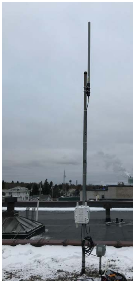
CGR and antenna on rooftop
