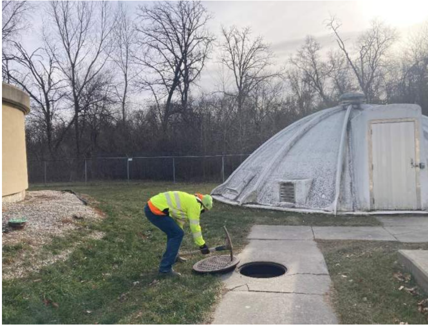
Photo 7 – View looking south showing Corey removing manhole lid of effluent manhole #2 with fiberglass dome of covered final clarifier #2 behind.
