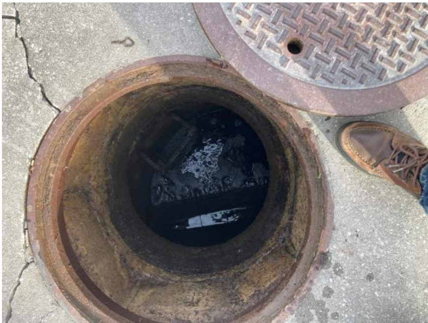
Photo 8 – View looking down inside effluent manhole #2 showing manhole steps and center weir wall.
