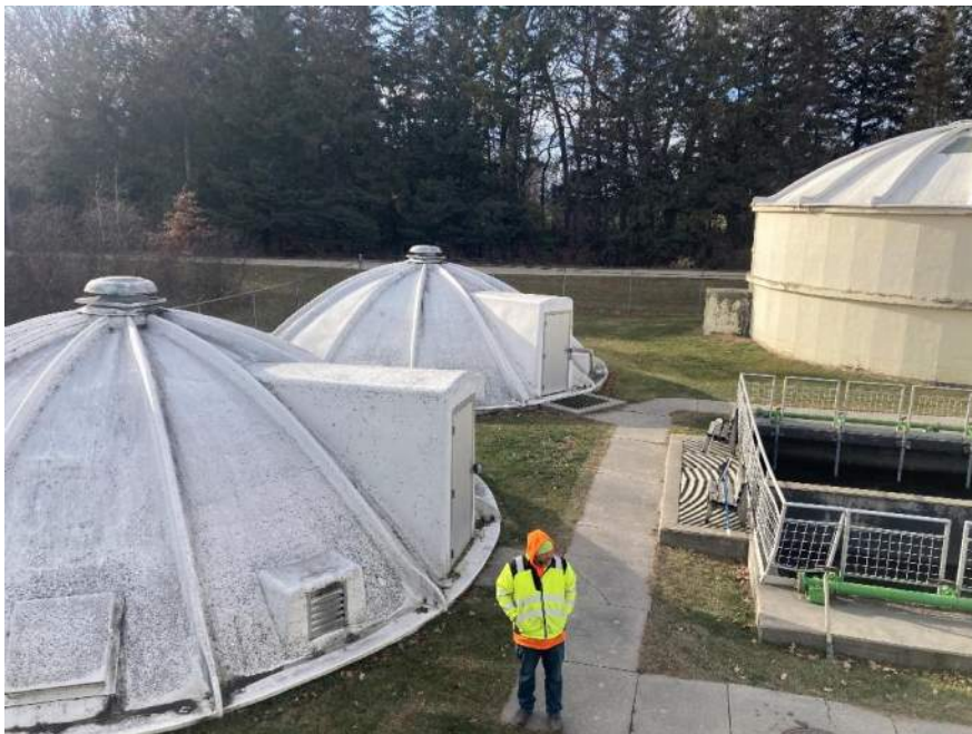
Photo 6 – View looking west showing both fiberglass dome covered final clarifiers #1 and #2
