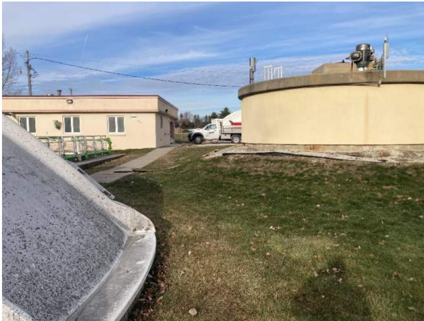
Photo 5 – View looking north showing tan colored concrete primary digester tank, pretreatment building, east side of fiberglass dome covered final clarifier #2, and effluent manhole #2 in sidewalk.
