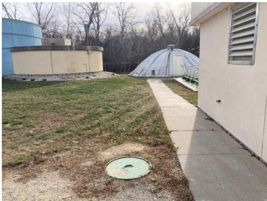
Photo 3 – View looking south showing effluent manhole #2 (green lid) in foreground and fiberglass dome covered final clarifier #2, primary digester concrete tank, and part of sludge storage tank (blue metal steel) upper left.
