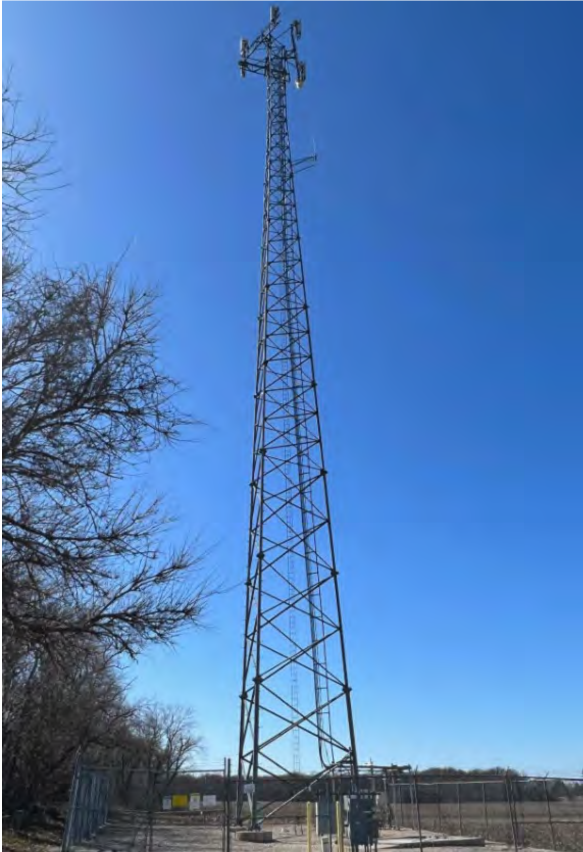
~200 foot self-support telecommunication tower
